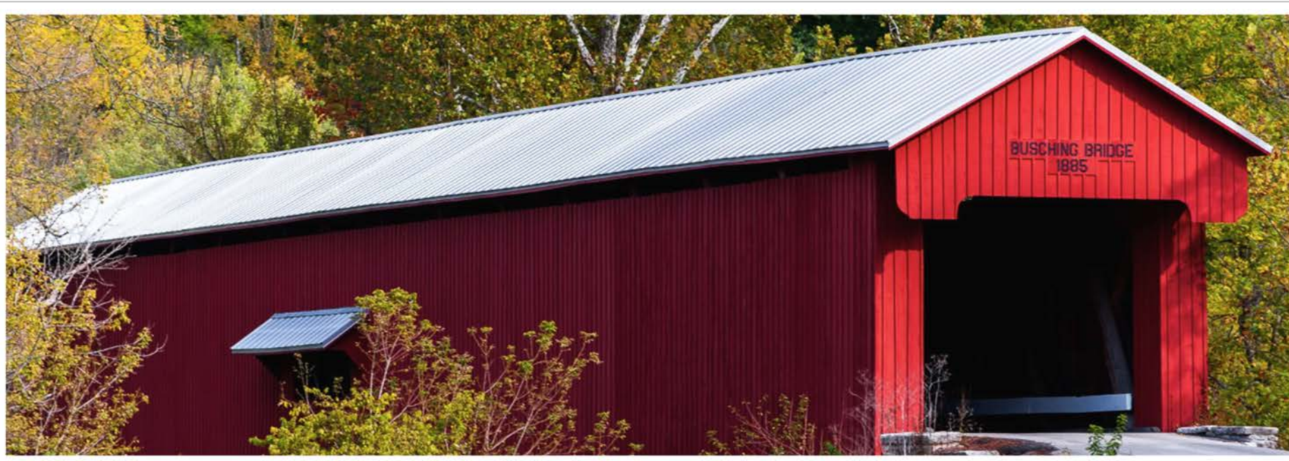
Busching Covered Bridge
